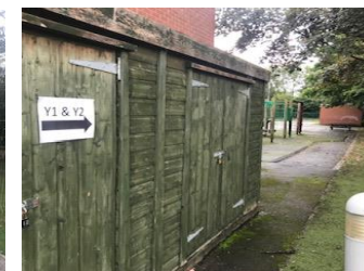
Pass sheds to classrooms.
